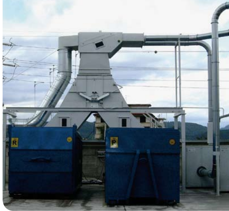
Scarico con By-pass pendolare Discharge system with switching By-pass
